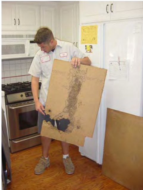
Mike finds Subterranean Termite Damage
