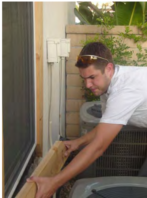
Mike replacing Drywood Termite window damage
